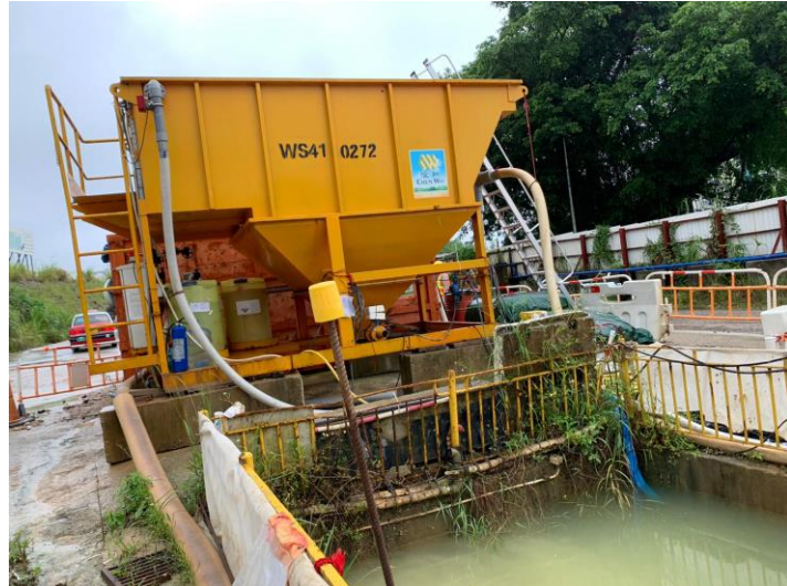
Q6: Wastewater treatment facility 24 cu. m.
