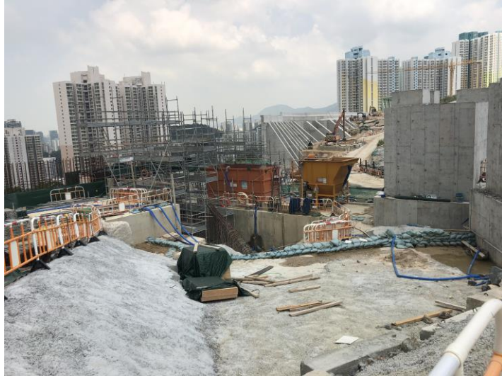
Paving for exposed slope to reduce dust dispersion & mitigate the silty runoff generation at SYSTEM A.
