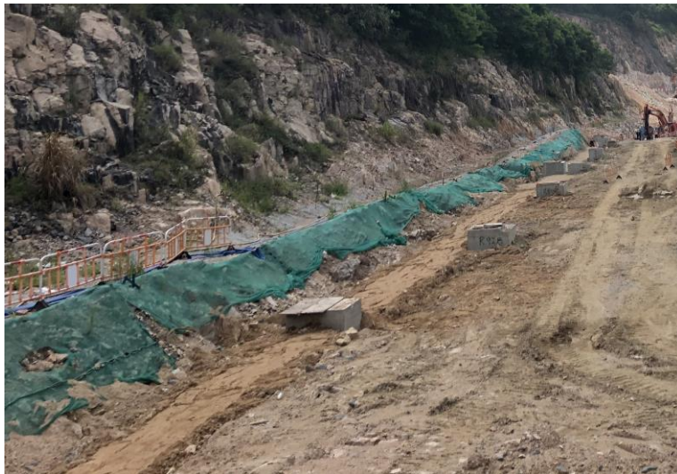
Impermeable cover for slope at PTT
