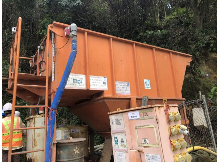
Q9. Two nos. of 30 cu.m Sedimentation Tank + AquaSed of 60 cu.m per hour
