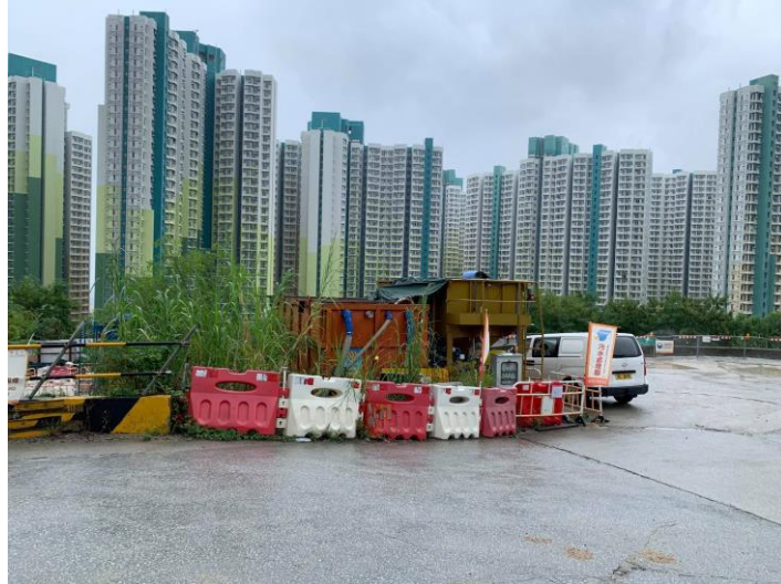
Q1. Wastewater treatment facility 30 cu.m Sedimentation Tank + AquaSed of 15 cu.m per hour
