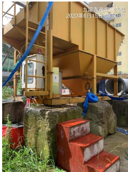
Q7. Wastewater treatment facility 30 cu.m Sedimentation Tank + AquaSed of 60 cu.m per hour
